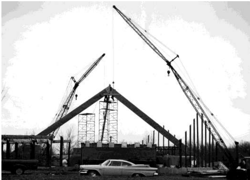
The construction of the current sanctuary. This sanctuary was dedicated on June 27, 1965.
